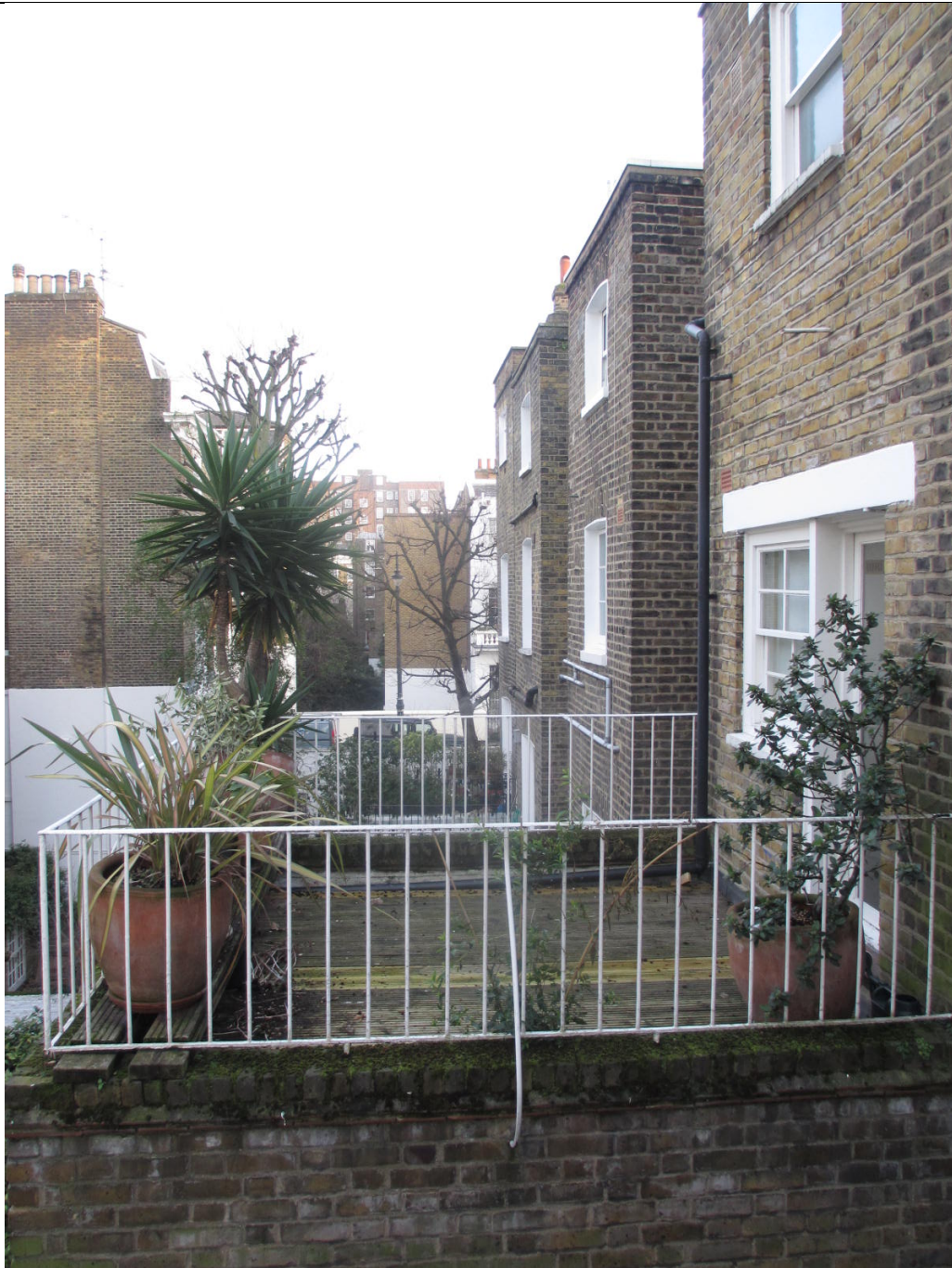
View of existing terrace next door at no.85 Alderney Street
