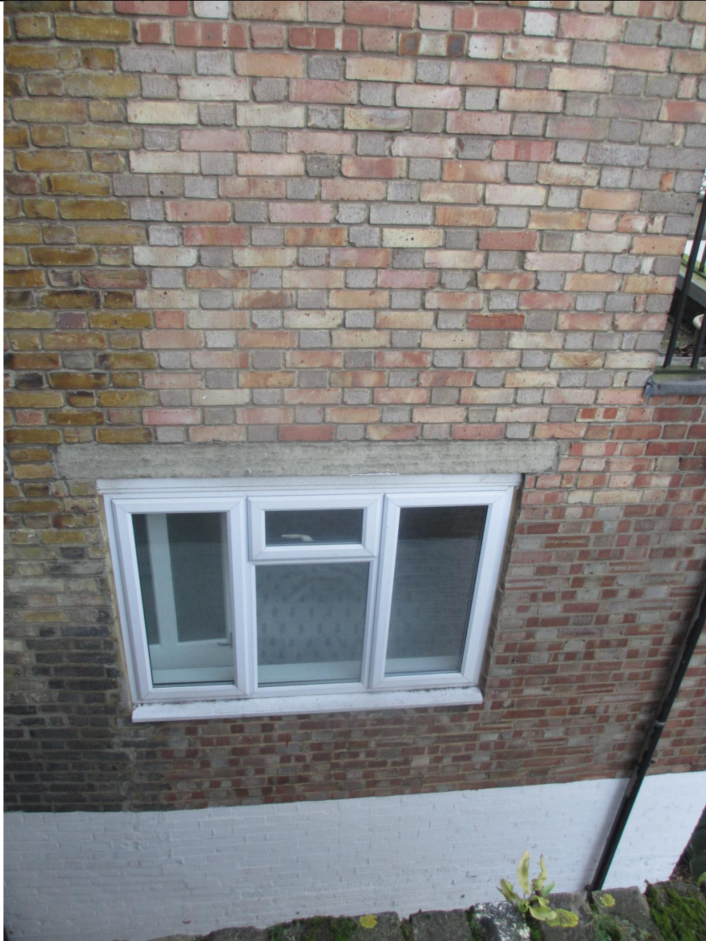
View of objectors' first floor bedroom window at no.81 Alderney Street
